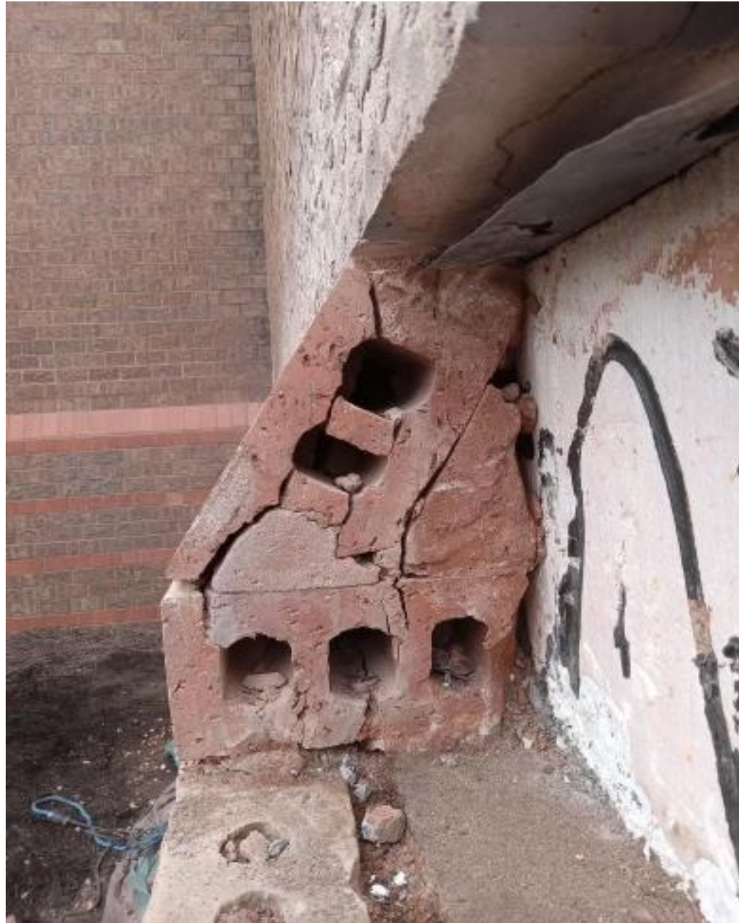
Church South Wall Brick Repair
