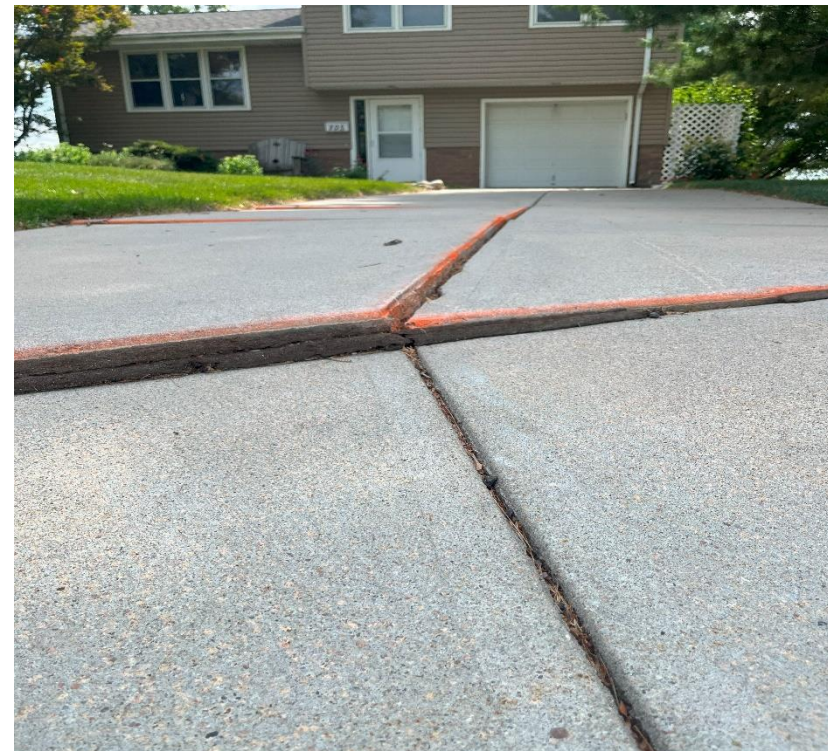
Concrete Repairs at the Rectories and School Campus
